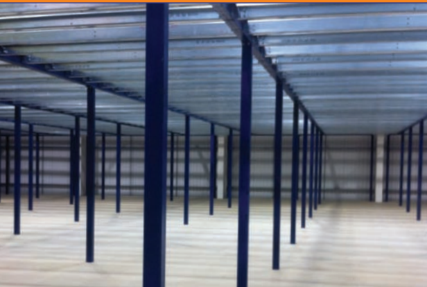
Another mezzanine floor under construction
